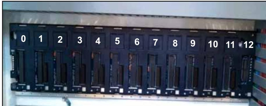
2. Install the new PLC power supply.
